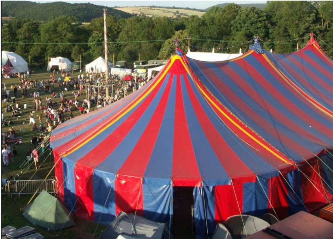
Roustabout's Big Top: 60' x 120' Three king-poles with 10' high side walls
