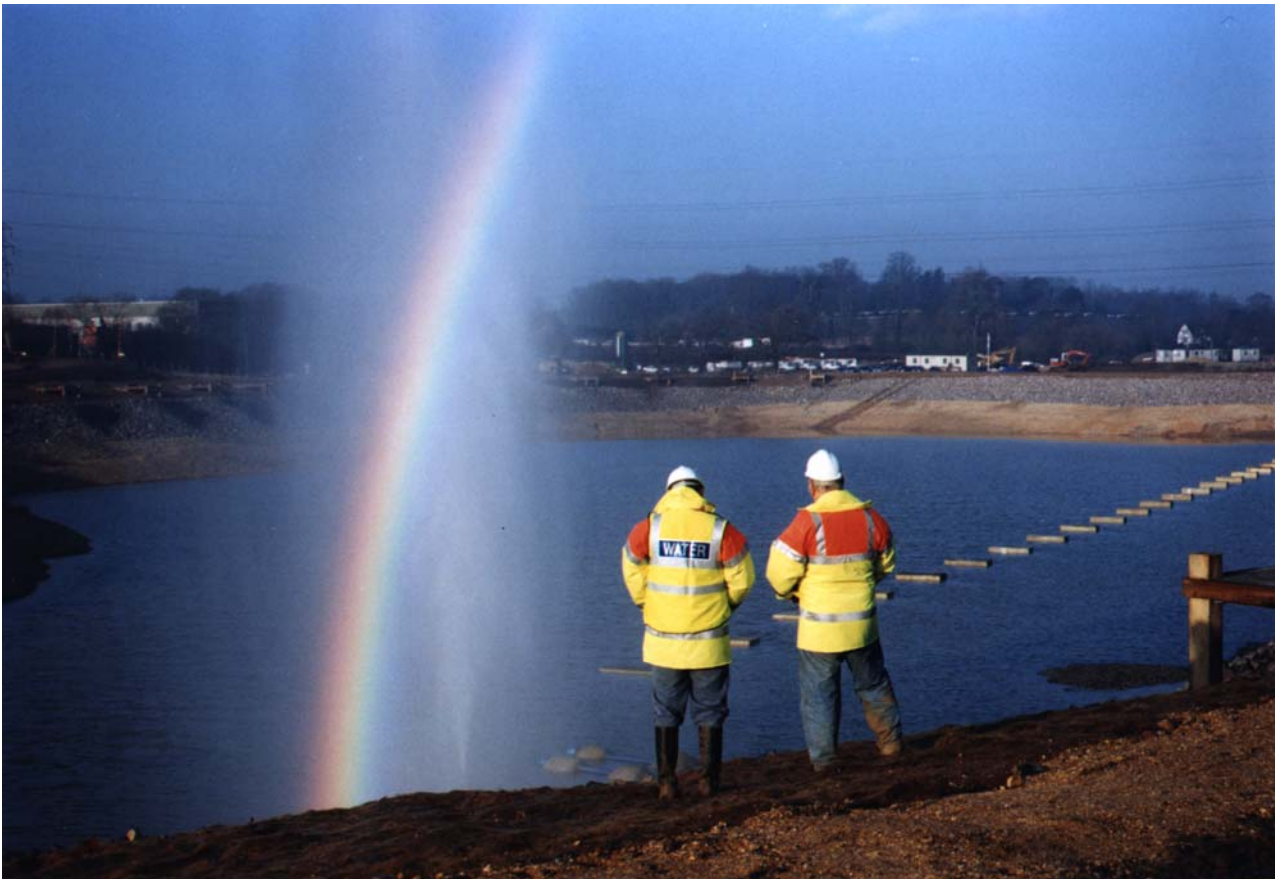
Adequate water resources are essential when planning a development
