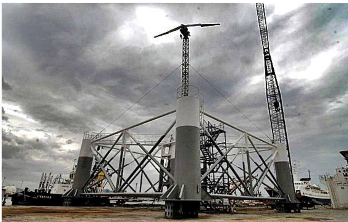
This photo is of the Hydriada experimental wind turbine for desalination being trialled in the Aegean Sea, Greek Islands
